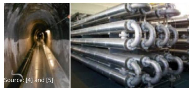
constructions, elements with factory-integrated heat exchangers can be used, thus exploiting cost synergies. The heat exchanger surfaces are made of a material with high thermal conductivity and are usually double-layered for the flow of an intermediate medium. The length of a heat exchanger can easily be 200-300 m [6].
