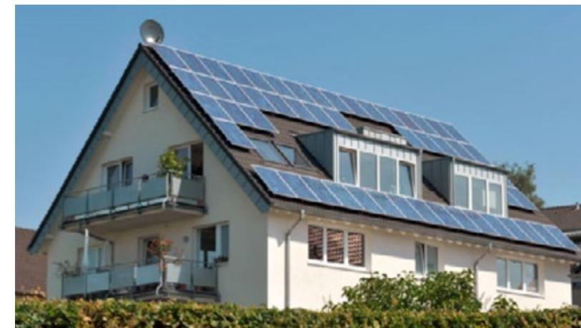
This multi-family house was built in 2011. There are seven flats with a total area of 541 m<sup>2</sup> occupied by 11 people. The air source heat pump delivers space heating through panel heating. Floor heating is used to distribute the heat in the building. The capacity of the heat pump is 22.4 kW and the annual COP is around 4.03. The heat pump was combined with PV modules, which leads to the best energy efficiency values in this case. Source [2]
