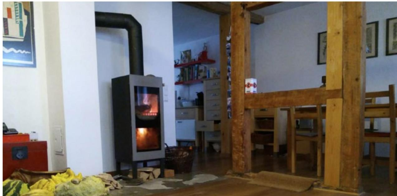
A typical application is this stove in a private single-family house (with a living space of 170 m<sup>2</sup>). The stove covers approximately 30% of the heat demand of the building. The rest is covered by a conventional heating system. The wood is delivered by a local biomass supplier and partly covered by private wood supplies. Essential for the twin-fire operation is dry and clean wood and an adequate ignition process of approximately 20 min.
