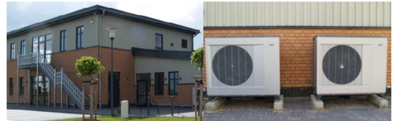
The fire station was built in 2014. Two air source heat pumps were installed for space heating and for domestic hot water. The heat is distributed through panel heating in the rooms. The rooms are supplied with three different temperature levels, which depend on the use schedule and the activities to be performed. There are PV modules on the roof to supply the accumulator, which is used to secure the electricity supply during blackouts. Source: [1]
